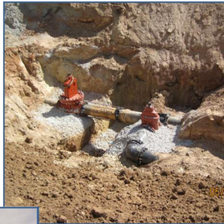
Tapping and relocating existing Water Line serving the GA Dome (above)
