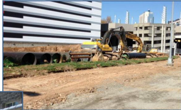
Jack and Bore Operation south of GA Dome for Sanitary and Storm Sewer (right)
